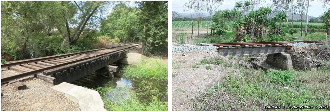
Figure 4.6: Steel Girder Culverts
