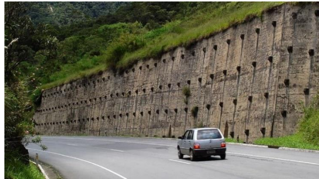
Figure 6.1: Typical Retaining wall
